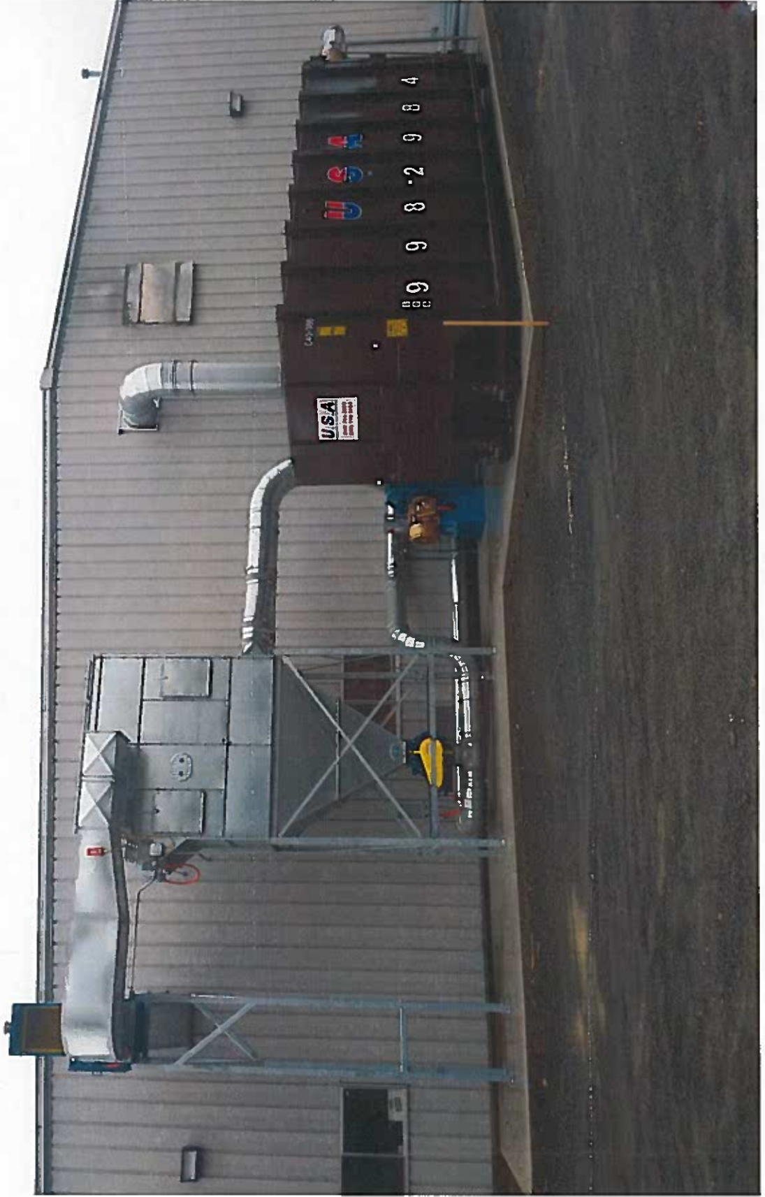
Example of Dust Collection System .
