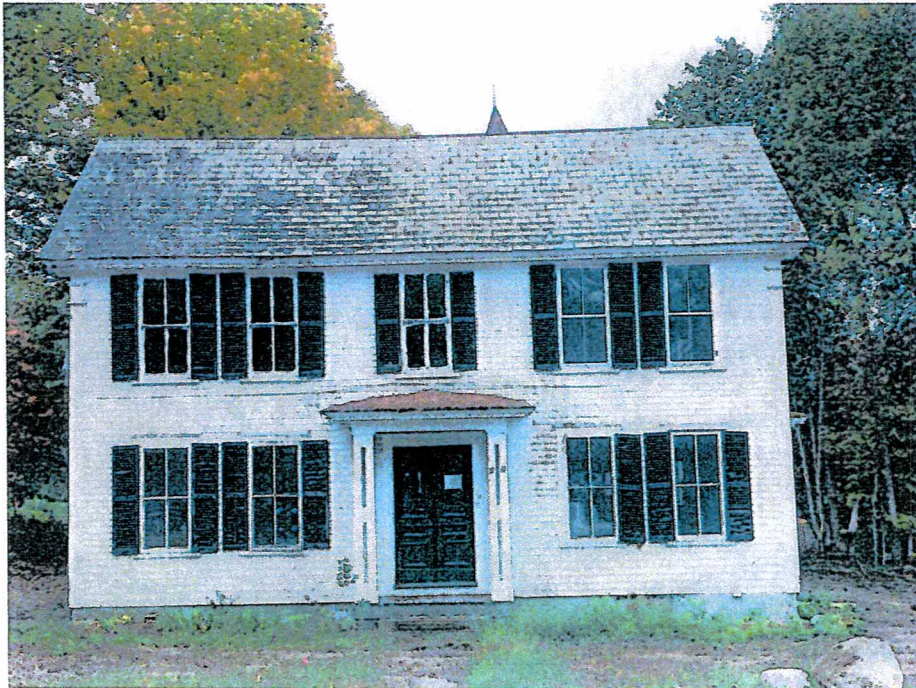
Front view of existing Building Picture taken 10/2018
