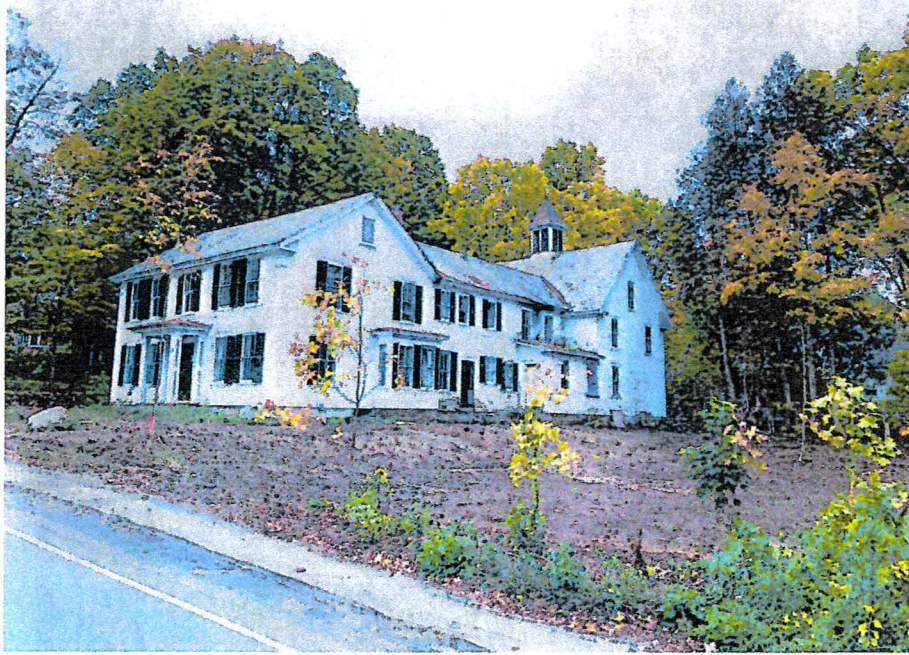
North side of the site Picture taken 10/2018
