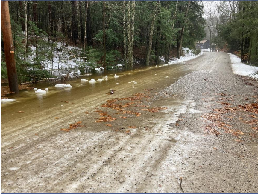
2022 Dec 23: Snowmelt Flood on Patch Road (CNHRPC)
