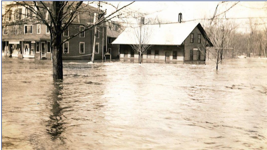
1936 March: Flood at Contoocook Flood Depot (Historical Society)
