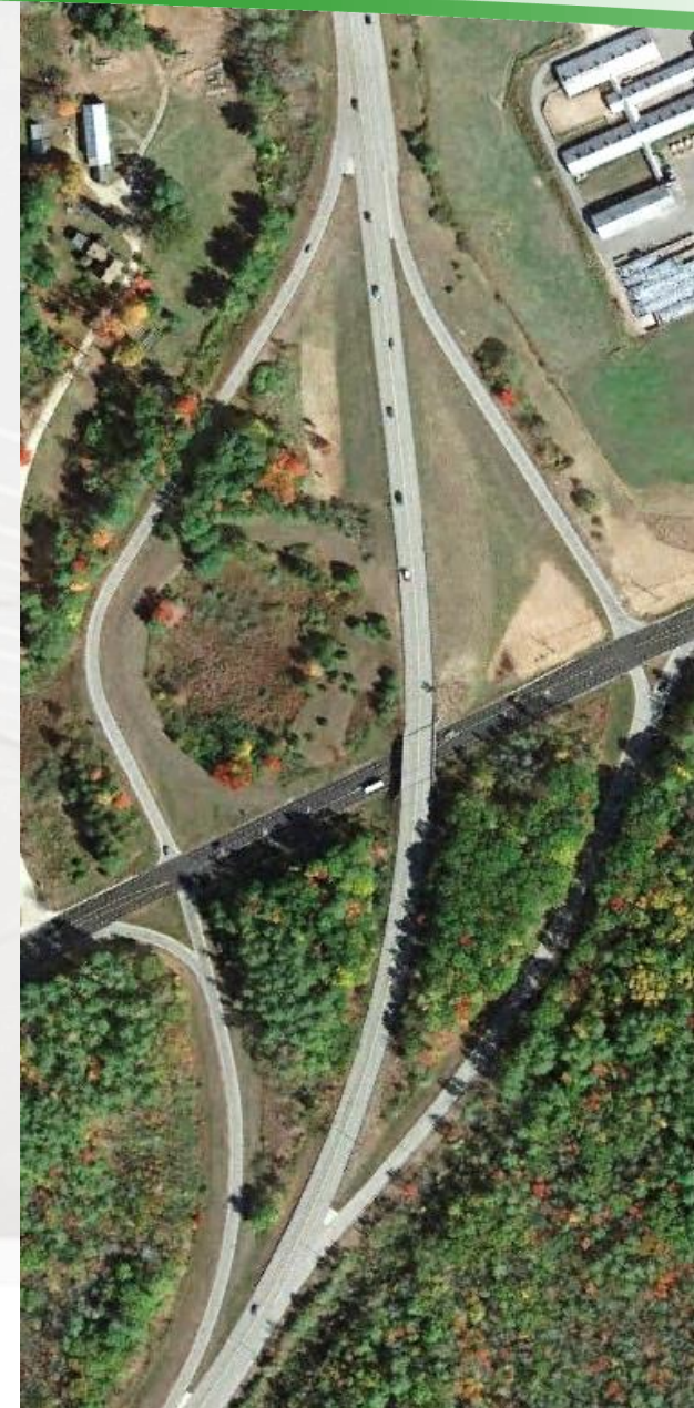
Image: Example grade separated interchange (US 4/NH 155A, Durham)
