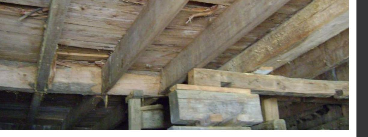
Northwest section of undercarriage, damage to floor and subfloor framing, temporary cribbing.
