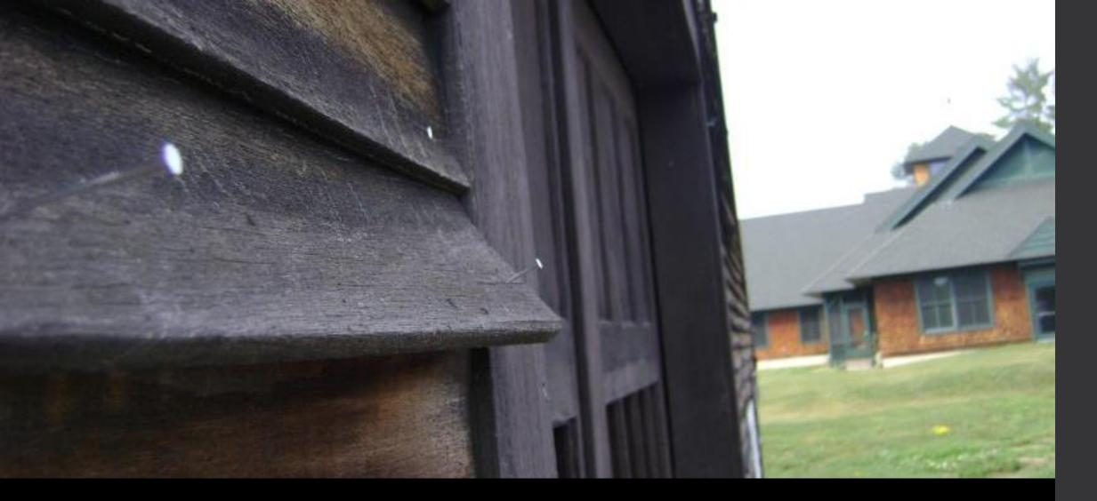
Clapboards warped and detached, with nails pulled. Typical of many.
