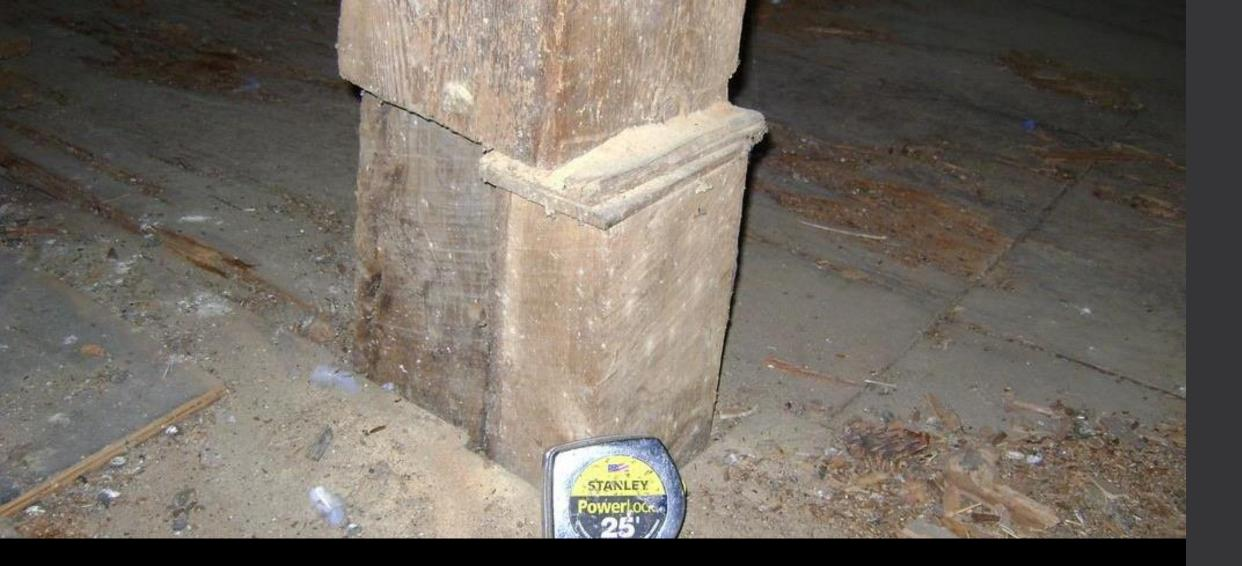
Post cut off and shimmed, also active insect boreholes and frass evident.
