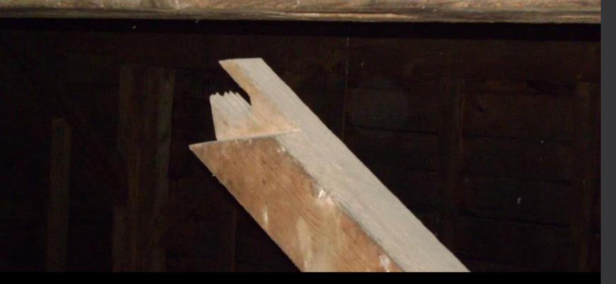
Disconnected knee-brace, indication of settling and distortion of major frame timers.
