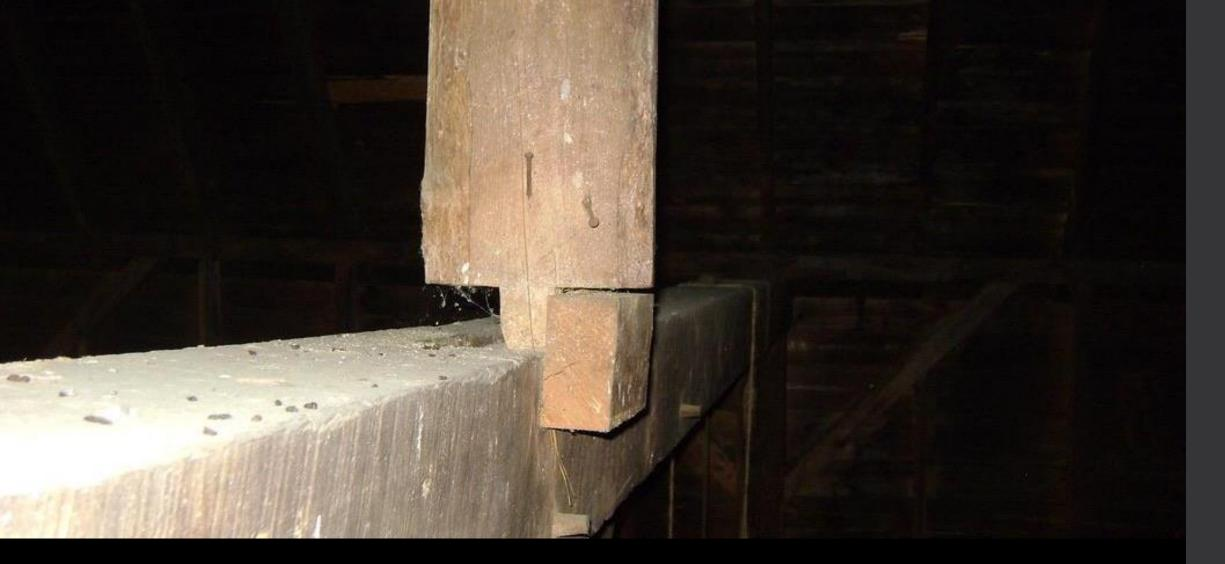
Displaced tenon at tie beam. Vital roof support is potentially compromised.
