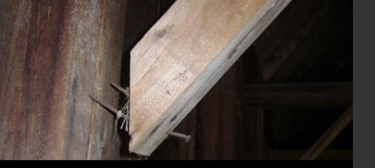
Nailed knee-brace connection at wall post separated.
