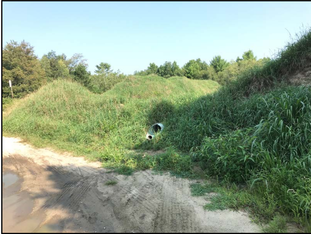
Photo #3 – Lagoon 1 Hauler Discharge Location (Looking North)
